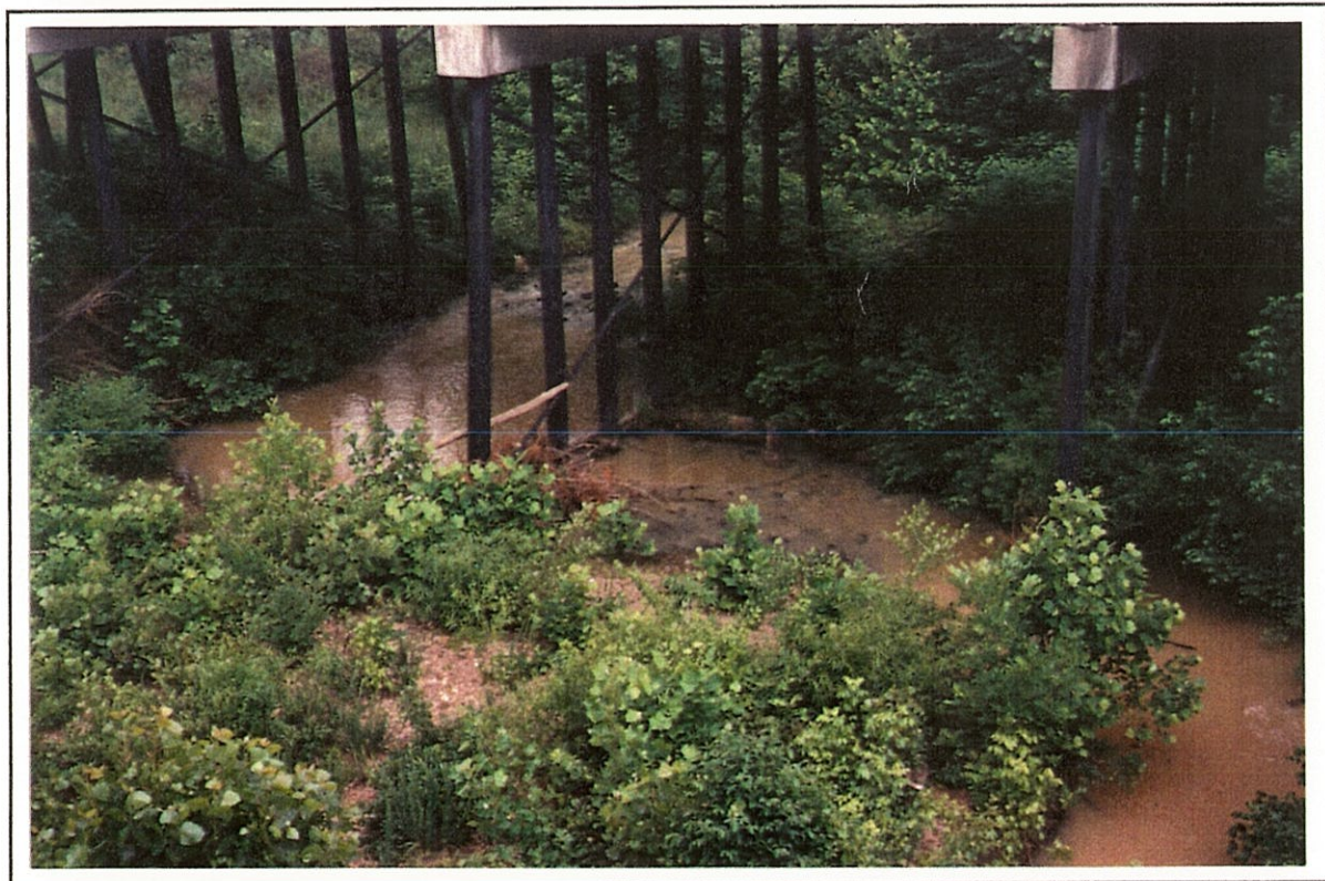
Figure 10. --Structure 121007730500 as viewed from structure 121007710500 on Interstate 77, crossing South Fork Fishing Creek in Chester County, South Carolina (note debris accumulation and sharp meander in low flow channel) (February 10, 1992).
